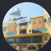
Fortis Hospital, Nagarbhavi, Bengaluru
