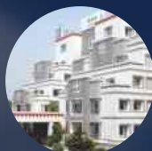
Fortis Hospital, Vasant Kunj, Delhi
