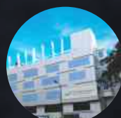
Gleneagles Hospital, Richmond Road, Bengaluru
