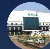
Fortis Hospital, Chandigarh Road, Ludhiana
